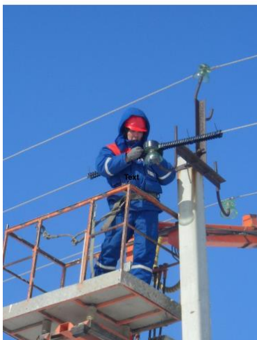
Installation of bird protection devices
